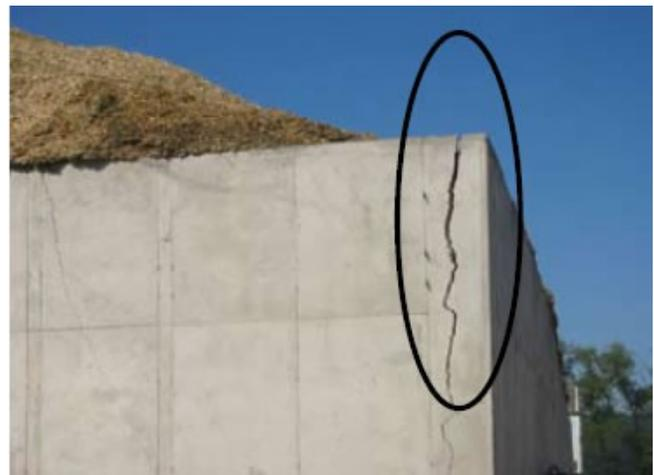
Figure 2. A cracked bunker sidewall needs repair.
